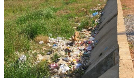
Rubbish at the creek near 6 th Street
