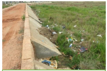
Rubbish at the creek near 6 th Street
